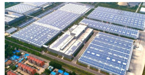
Distributed PV applications in industrial and commercial
