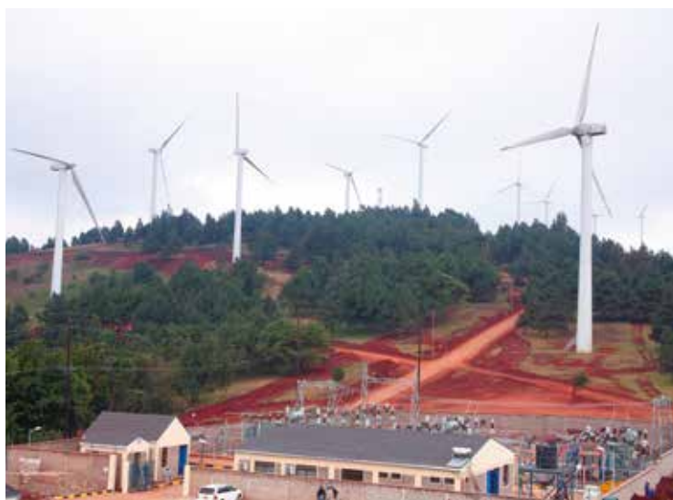
KenGen Ngong Wind Power Station, Kenya
